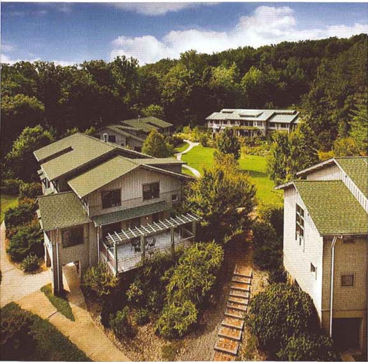
LEFT: The EcoDorm at Warren Wilson College (far center) is the fourth in the series of Ballfield Dorms. The EcoDorm is certified LEED-EB Platinum, the first such designation for a dormitory in the United States. All photos: John Warner, courtesy of Samsel Architects
